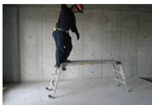
Moving up and down a scaffold ladder
